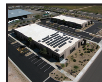
Integrity Building Corporation - Mesa, AZ 19.2kW System Performing at 106%
